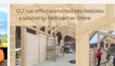
CLT cut-offs transformed into Rebloks – a solution by RAW partner Omtre
